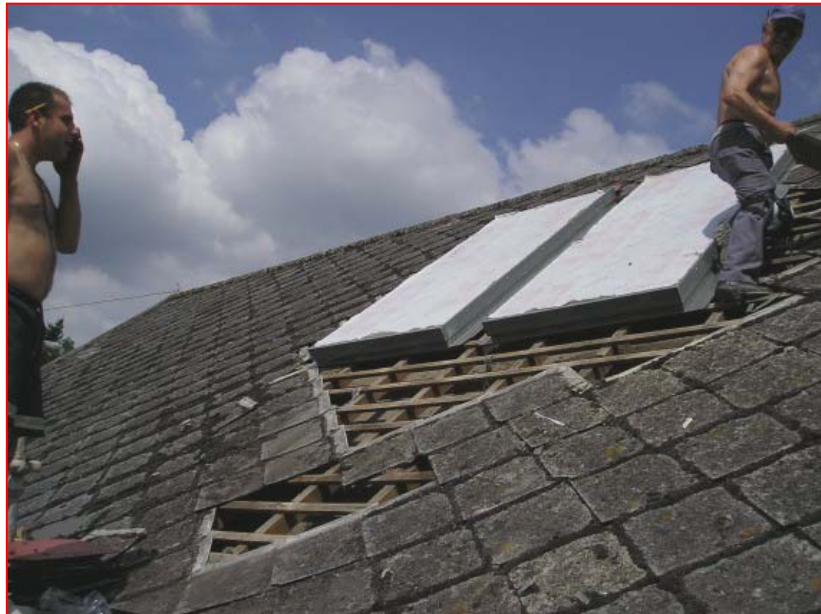
Installation during roof overhaul
