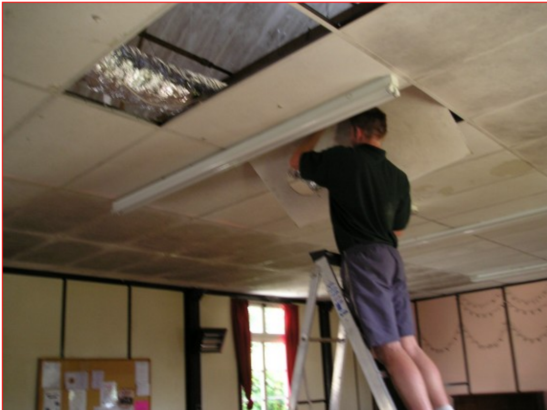
Installing Heat Recovery Ventilation
