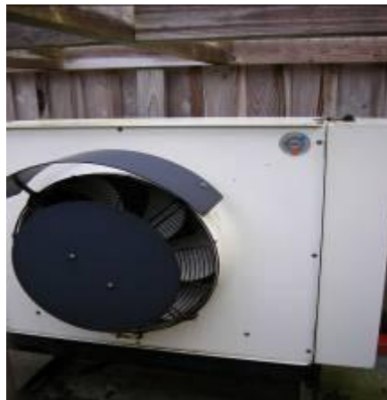
Air source heat pump, Barra learning centre
