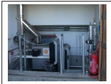
Typical wood chip boiler and hopper
