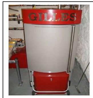
Wood pellet hopper and boiler
