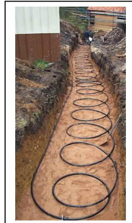
Examples of sinking a borehole (vertical loop) and a 'slinky' cable (horizontal loop) for Ground source heat pumps.
