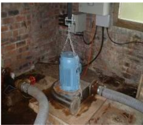
The turbine for Eigg pier hydro
