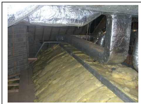
Typical loft insulation and pipe lagging
