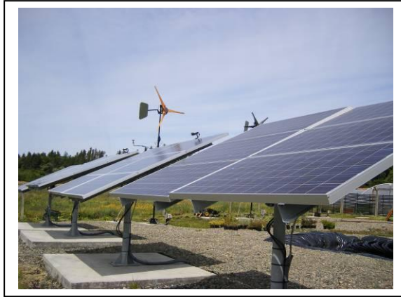
Ground mounted PV panels
