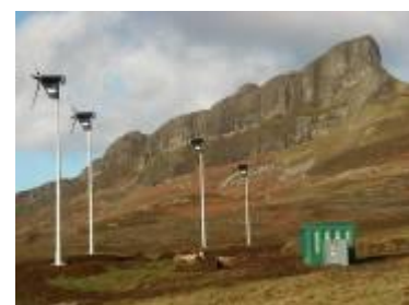
Four 6kW Proven turbines, Eigg electrification
