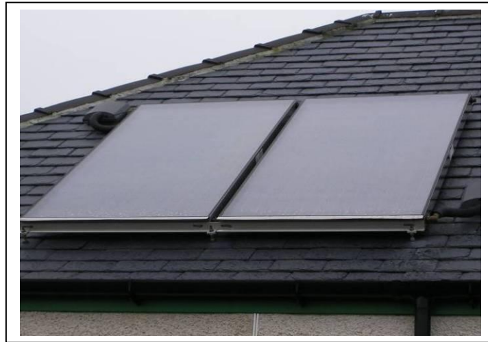
Flat plate collector solar water heating panels
