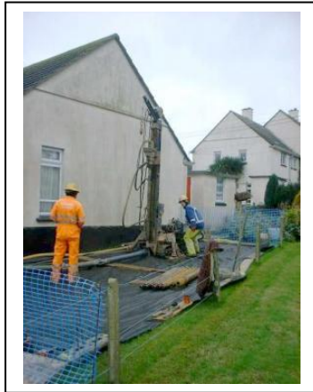
Examples of sinking a borehole (vertical loop) and a 'slinky' cable (horizontal loop) for Ground source heat pumps.
