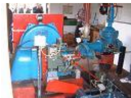
Gilkes & Gordon 350KVa pelton turbine
