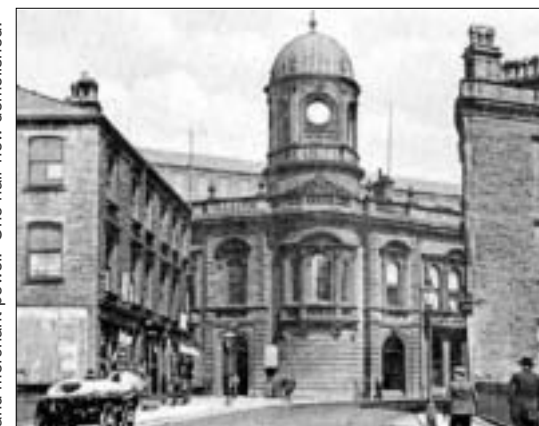
Town Hall, Sowerby Bridge, a statement of civic and merchant power. One half now demolished.
