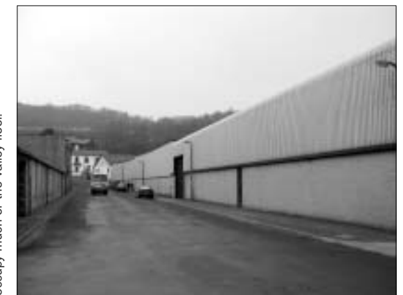
Large footprint, single storey industrial sheds now occupy much of the valley floor.
