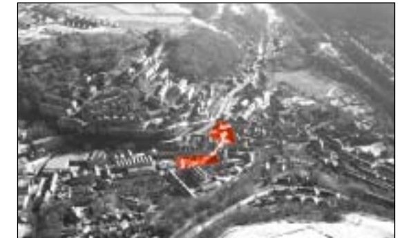
Reinforcing the Heart of the Town
