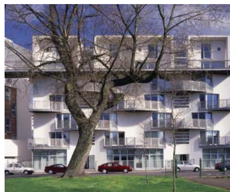
FIGURE 4.9 Glasgow housing, Rick Mather Architects
