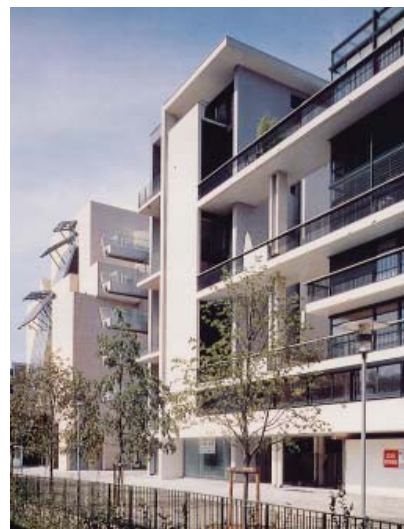
FIGURE 4.10 Facade demonstrating the potential of large balconies and fenestrations
