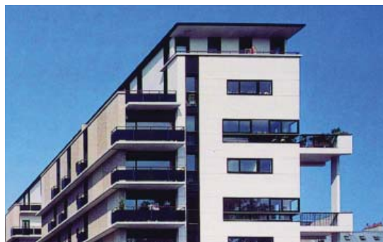
FIGURE 4.12 Example of external balconies and terraces
