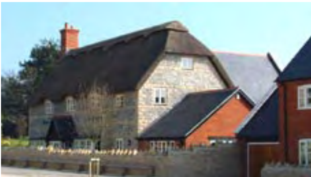
Houses set back a maximum of 2m from back of pavement on a typical residential street
