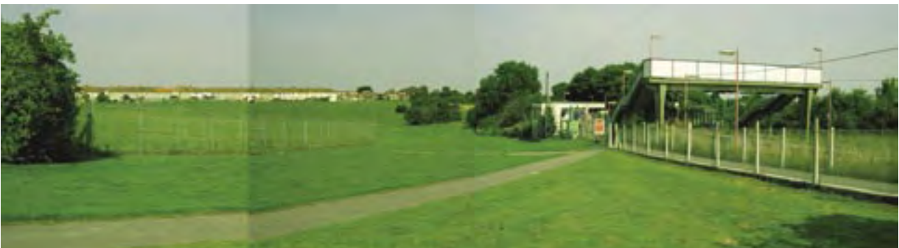
Poor pedestrian access to Aylesham station
