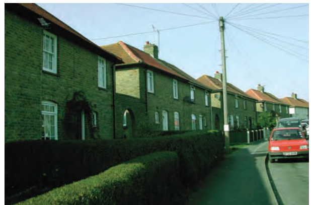
Original Abercrombie buildings
