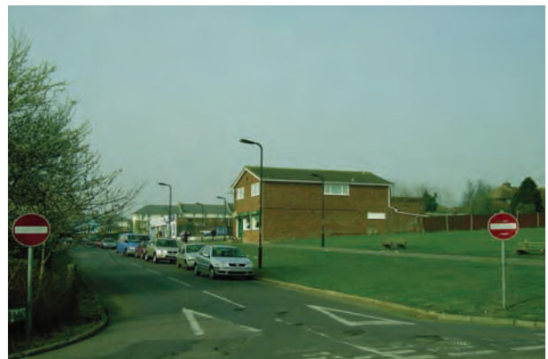
Existing Post office buildings
