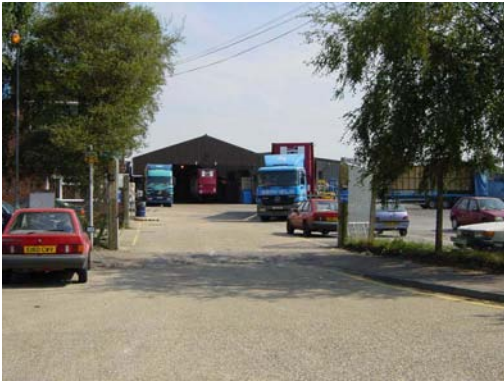
Aylesham Industrial Estate
