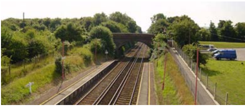
Aylesham Station, looking south
