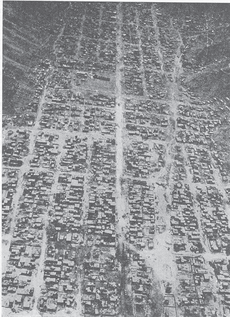
1961 — Dense provisional encampment houses settlers while plans are being made for this site
