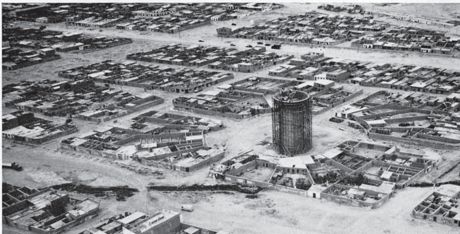
Below: the San Martín barriada—a reservoir under construction (left), and the installation of water and sewer mains in a street
