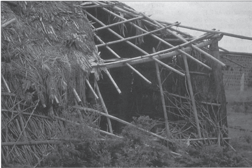
Flimsy structures cannot withstand cyclones.
