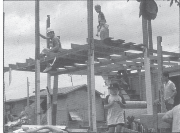
After land-sharing: dismantling a building for re-assembling on a new site.
