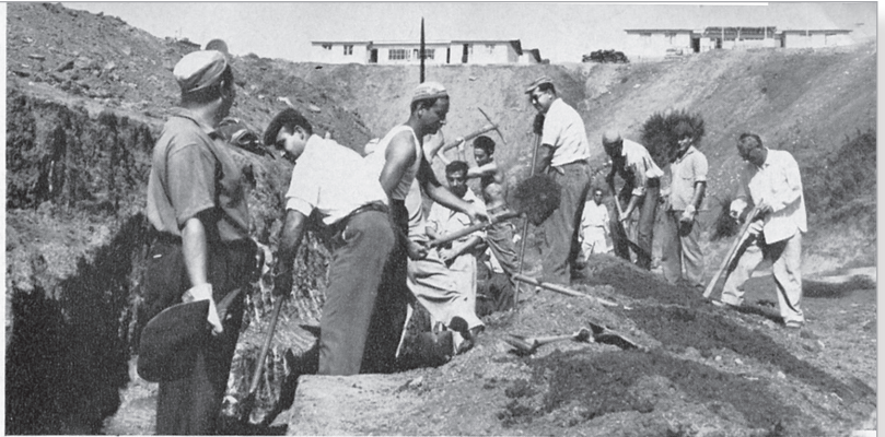
Above : owner-builders preparing the site for one of the houses
