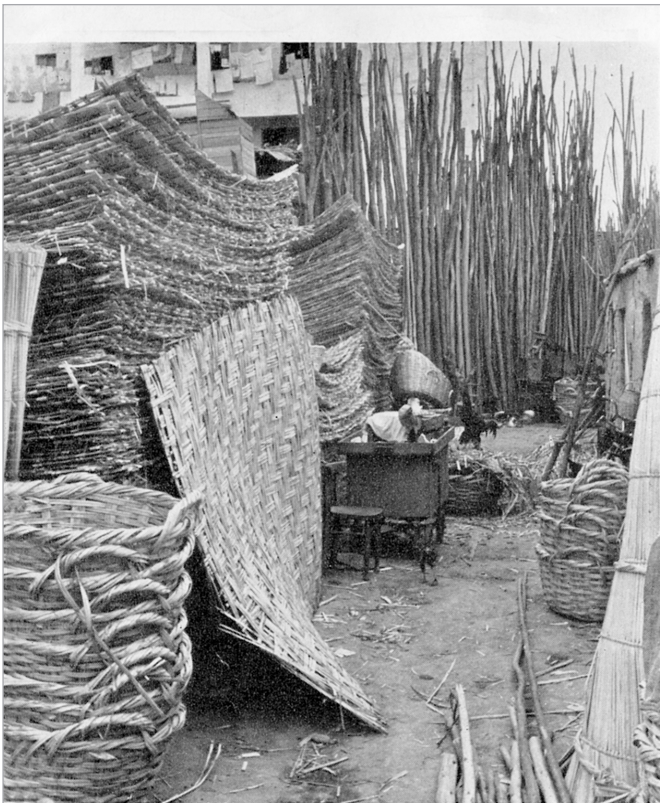
Above: sales yard for Lima 'barriada' house elements; mats and poles for the structure Photo William Mangin
